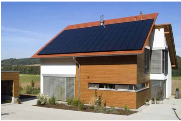
POWERline photovoltaic system with GeneCIS-modules from Würth Solar (Source: Würth Solar)
