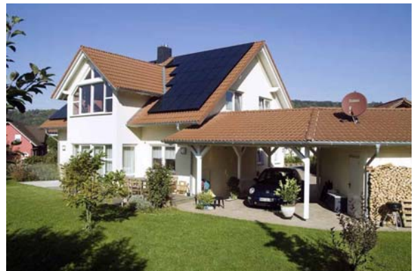
HOMEline photovoltaic system with GeneCIS-modules from Würth Solar (Source: Würth Solar)
