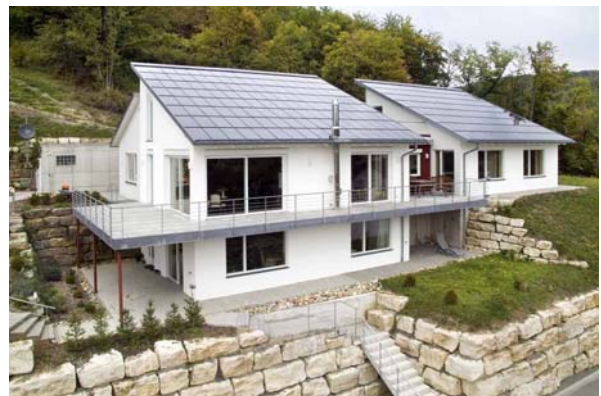
DESIGNline photovoltaic system with GeneCIS-modules from Würth Solar (Source: Würth Solar)
